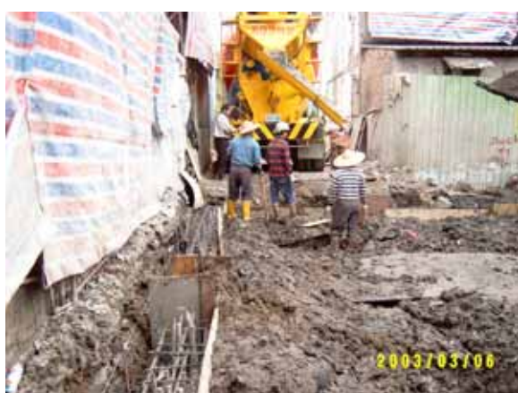
澆置壓樑混凝土
