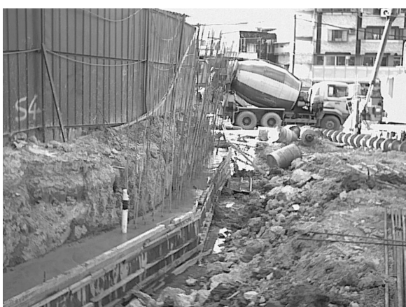
澆置壓樑混凝土
